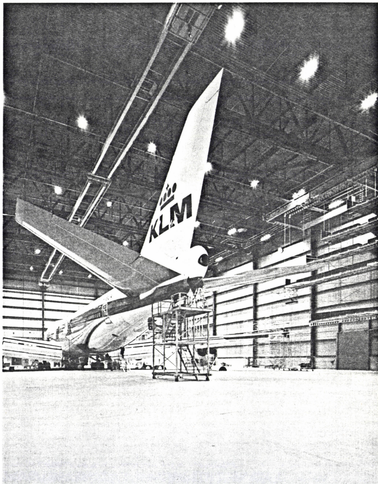
One of the three bays of the 'Jan Dellaert' hangar at Schiphol (Amsterdam Airport), specially built for maintenance work on Boeing 747 B aircraft. Each bay is illuminated by 199 high-pressure sodium lamps (400 W).
