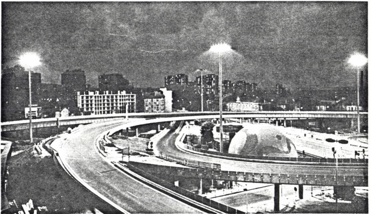
A traffic intersection in Cherbourg, illuminated by 96 metal-iodide lamps (HPIT 1000 W). The average illuminance at the road surface is 60 lux.
