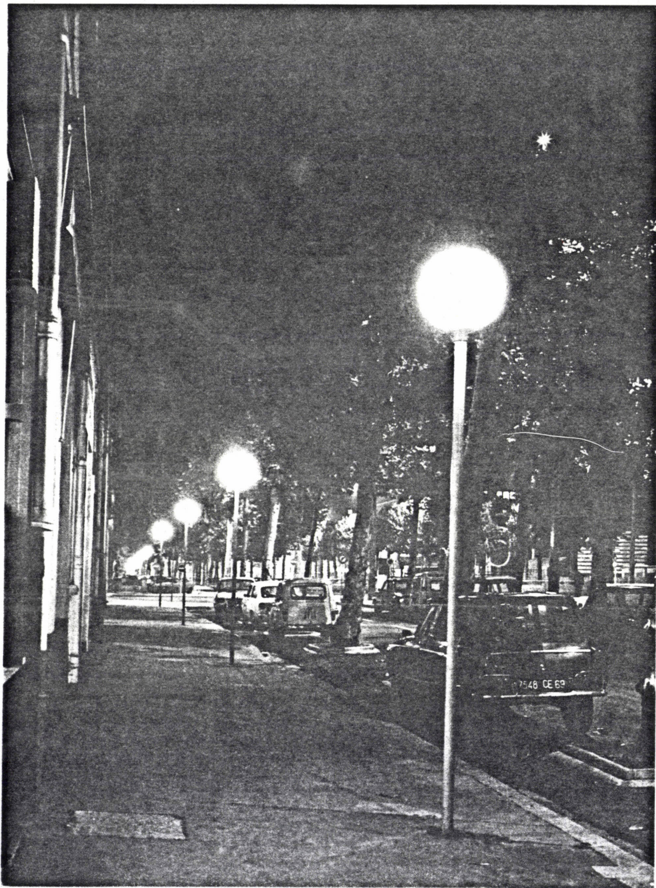
A street in Lyons (La part Dieu), illuminated at the centre by high-pressure sodium lamps (400 W) and along the pavements by high-pressure mercury-vapour lamps with fluorescent envelopes (125 W).
